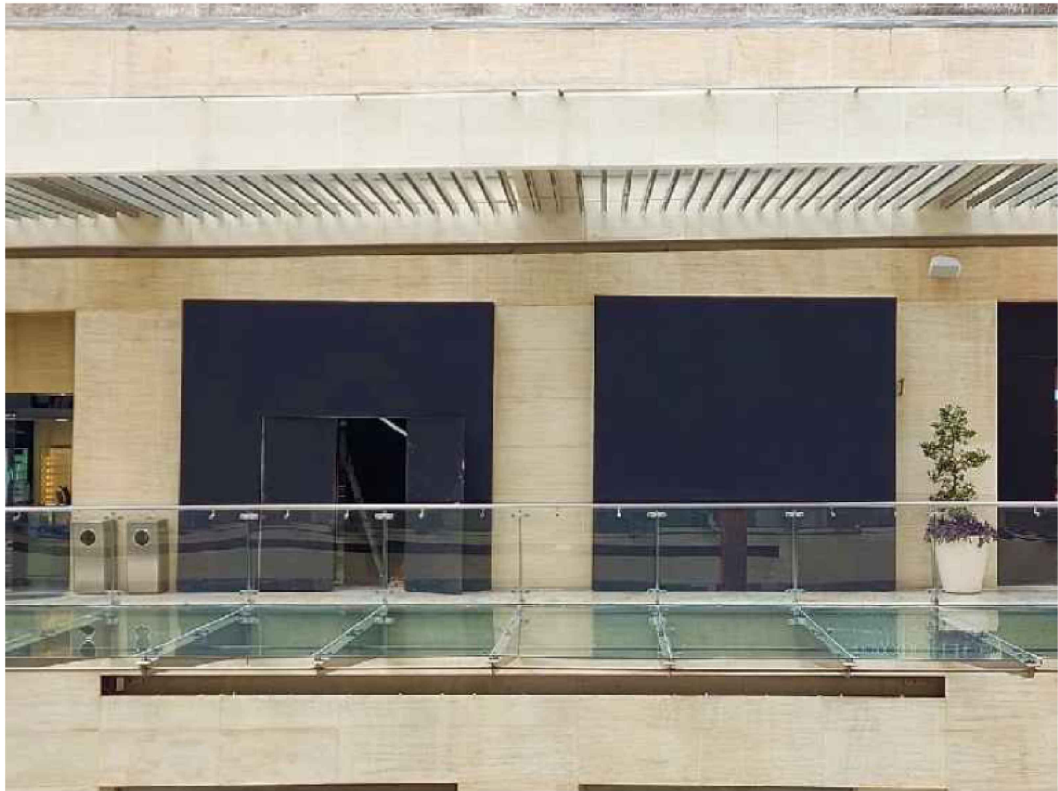
ESTADO ACTUAL DE FACHADA CURRENT STOREFRONT (WITH MUDWALL)
